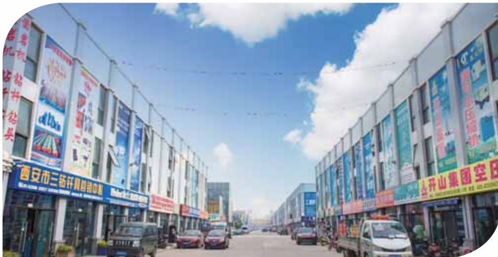
Hardware & machinery product trade center in trial operation 試運營中的五金機電交易中心
